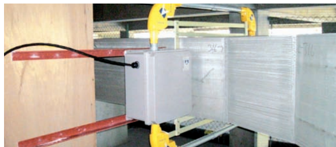
Dynamp 225 kA 0.1% class DC CT for aluminum smelting
